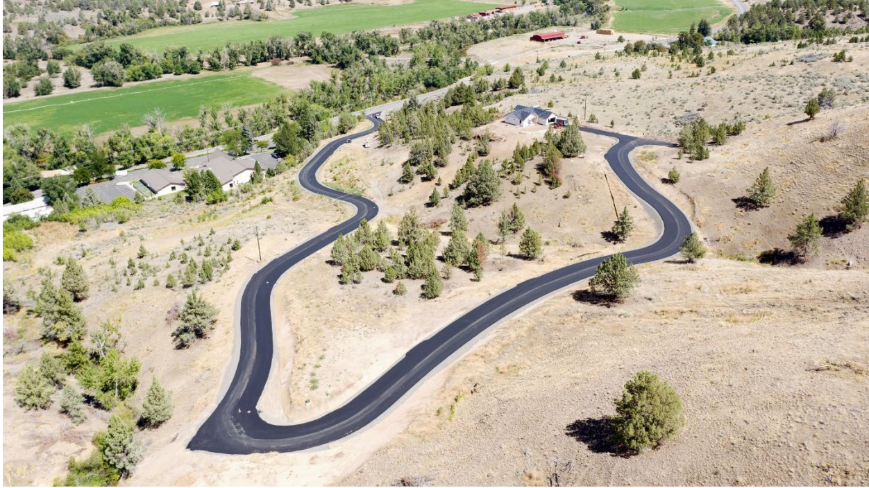
Figure 1. The Ridge, Phase 1
