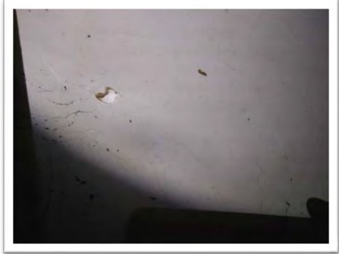
Sample 20-045A.12, Wall Materials, <1% Asbestos
