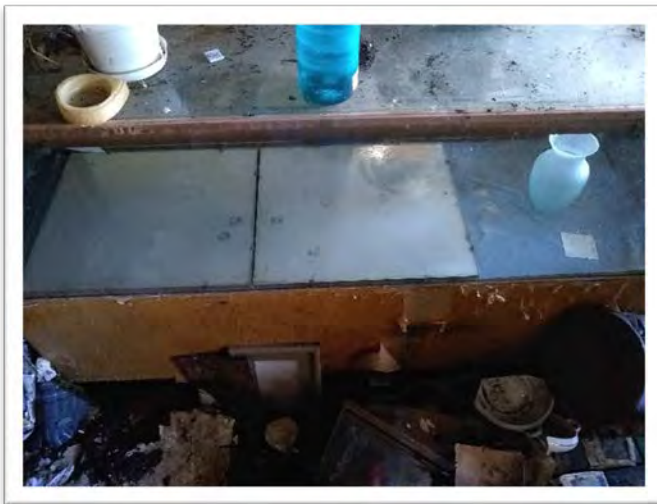
Sample 20-045A.L9, Yellow Paint, 700 ppm Lead
