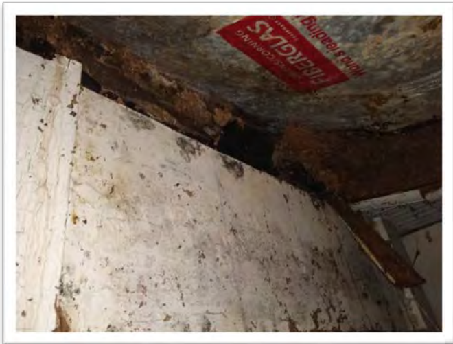
Sample 20-045A.25, Tar Paper, Non-ACM Sample 20-045A.26, Tar Paper, Non-ACM
