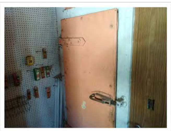
Sample 20-045A.L6, Orange Paint, 12,000 ppm Lead
