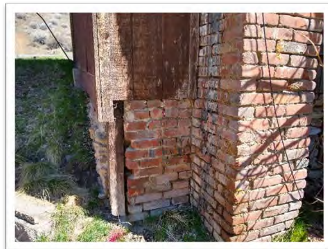
Samples 20-045A.37, 38, Red Brick, Non-ACM Samples 20-045A.39, 40, Mortar, Non-ACM
