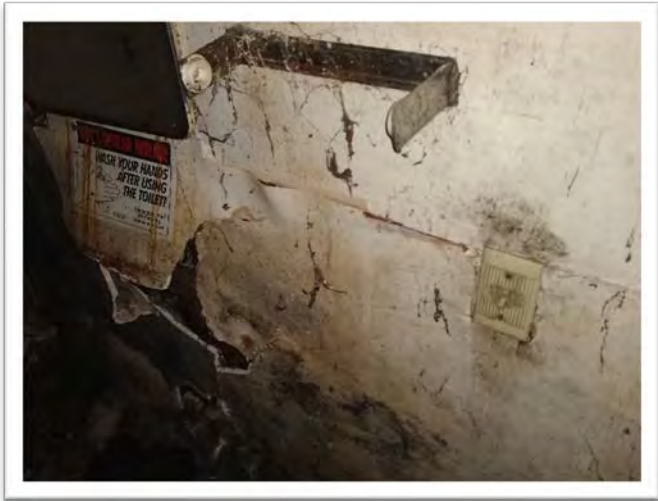
Sample 20-045A.11, Wall Materials, <1% Asbestos
