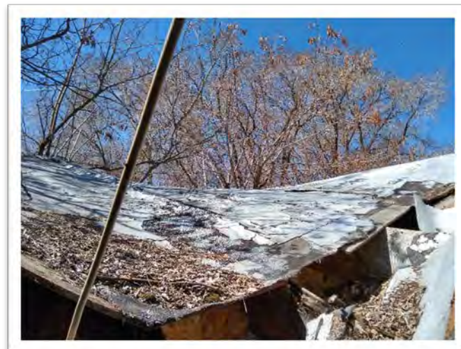
Sample 20-045A.23, Built-up Roof, <1% Asbestos
