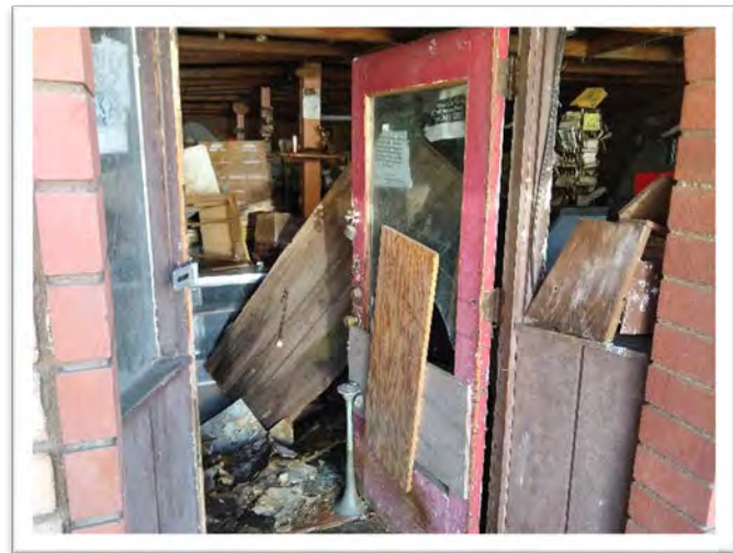
Sample 20-045A.L10, Red Paint, 16,000 ppm Lead
