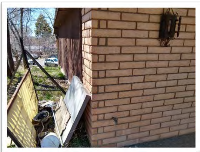
Sample 20-045A.34, Tan Brick, Non-ACM Sample 20-045A.36, Mortar, Non-ACM
