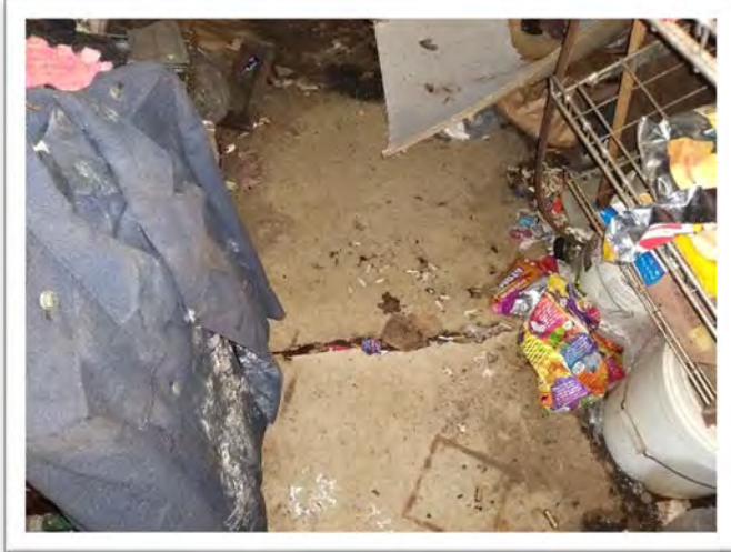
Sample 20-045A.2, Vinyl Floor, 20% Asbestos
