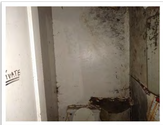
Sample 20-045A.13, Wall Materials, <1% Asbestos Sample 20-045A.14, Wall Materials, 2% Asbestos
