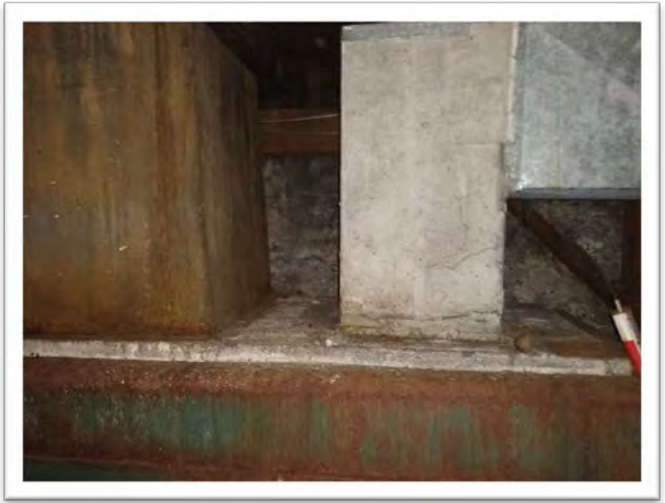
Sample 20-045A.44, Furnace Insulation, 40% Asbestos
