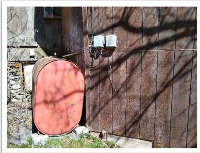
Sample 20-045A.L3, Brown Paint, <82 ppm Lead
