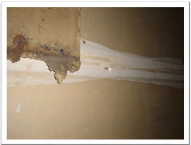
Sample 20-045A.47, Drywall/Mud, Non-ACM
