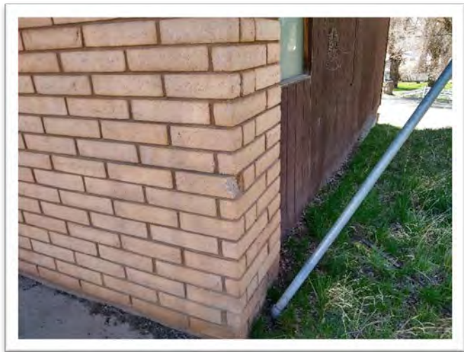
Sample 20-045A.33, Tan Brick, Non-ACM Sample 20-045A.35, Mortar, Non-ACM
