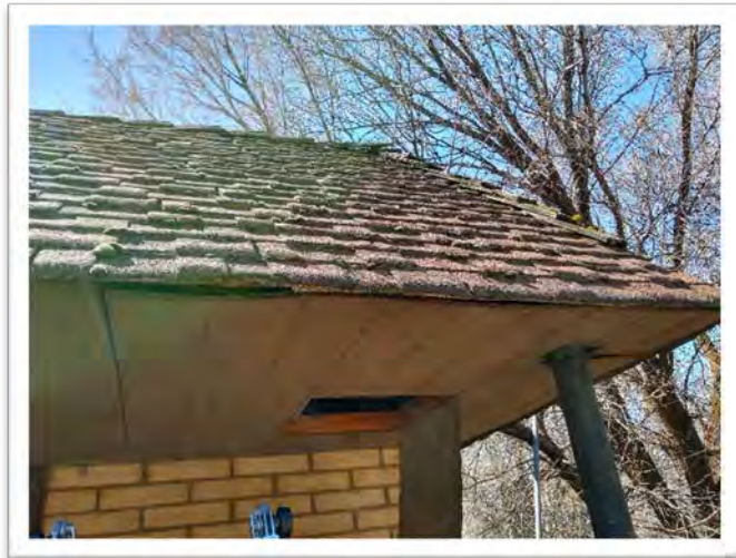
Samples 20-045A.27, 29, 31, Roof Layers, Non-ACM
