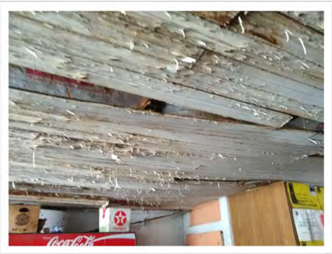
Sample 20-045A.L4, White Paint, 3,300 ppm Lead
